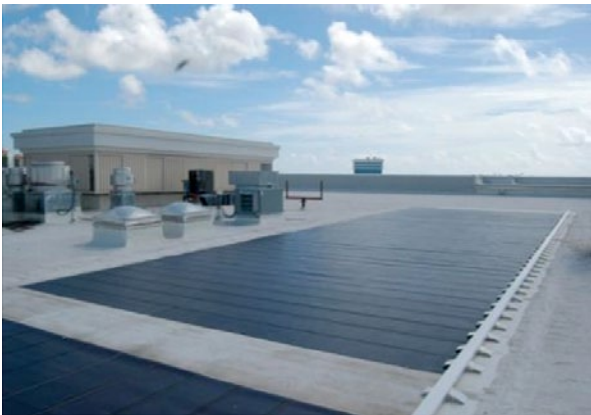
Thin film modules mounted on a flat roof. This flat-roof type is generally less efficient and requires more roof area than a sloped system. Source: Florida Solar Energy Center
